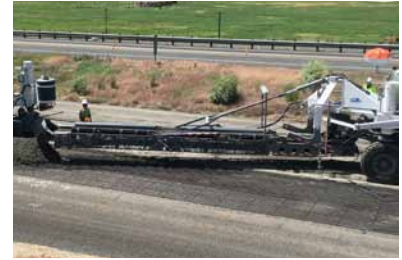
Hinging Swing Conveyor. 35' (10.7 m) Long 170 Degree Swing Arc
