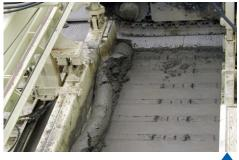
An Oscillating Correcting Beam, which is part of the DBI System, ensures accurate refinishing of the concrete surface disturbed by the dowel bar insertion process.
