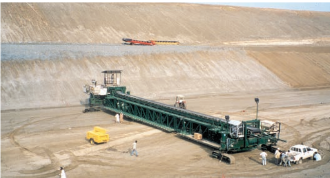
Half Span Liner in the canal bottom after counter-rotation. Patented Anti-torsion control protects the Liner latticework frame for potentially destructive torsional forces while walking over uneven ground.
