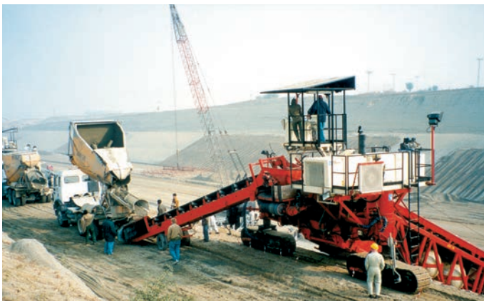
Agitator truck discharging into a charging conveyor.
