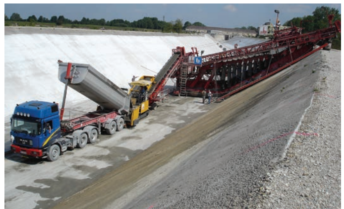
Semi-end Dump Trailer feeding a Concrete Placer.
