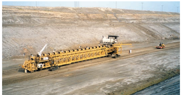
Half Span Trimmer walking and steering in along the canal bottom in the 90 degree steering mode under its own power.
