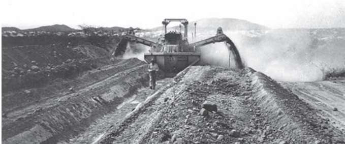
G&Z Canal Liner traveling on rails paving a canal bottom in Los Angeles, CA USA (1957).
