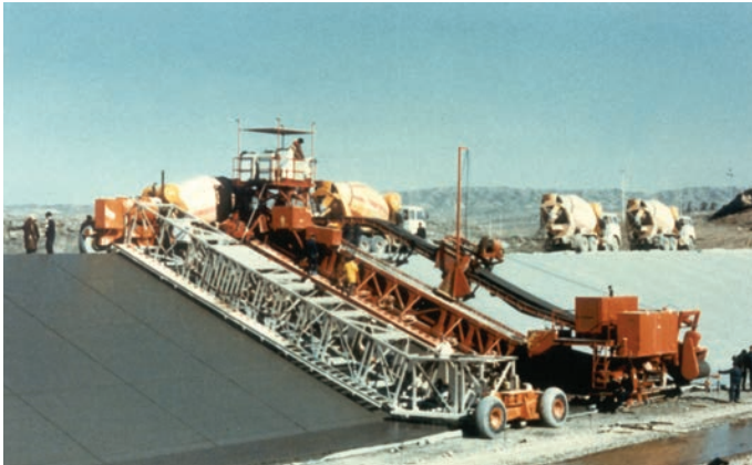
Two trucks discharge in a wiper conveyor.
