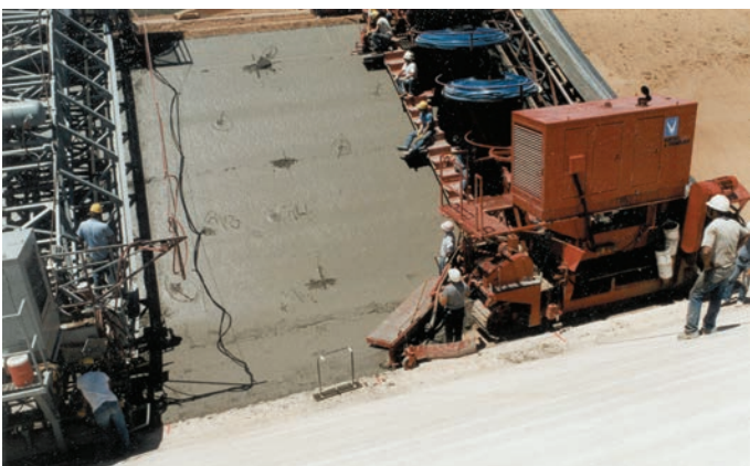
▲ Automatic longitudinal joint inserters for inserting PVC cruciform shaped water stop (blue material on reels).
