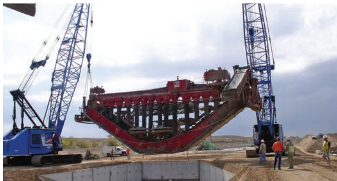
Two large cranes moving a full span canal liner over a structure in the canal alignment.
