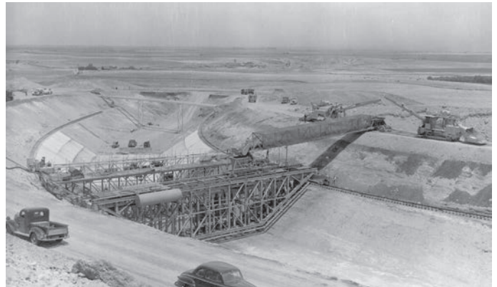
Rail mounted G&Z Canal Trimmer (top of page) and Canal Liner (above) (1947) working on the Delta Mendota Canal Project in California, USA.
