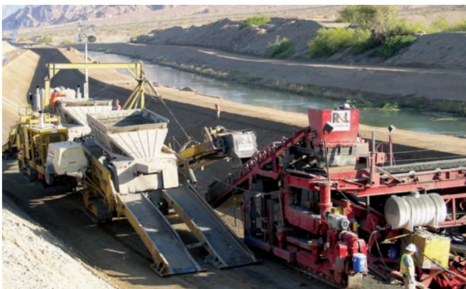
Tandem Belly Dump Trailers discharging from a crawler track mounted Drive Over Unloader.
