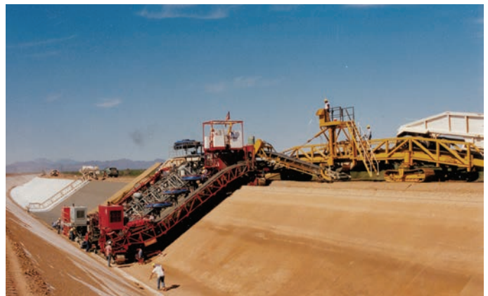
Semi Belly Dump Trailer discharging into a crawler track mounted Drive Over Unloader.
