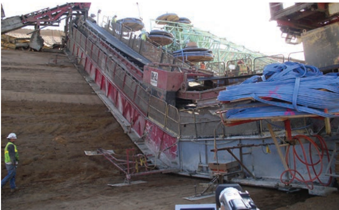
▲ Subgrade guidance ski for elevation and steering control.
