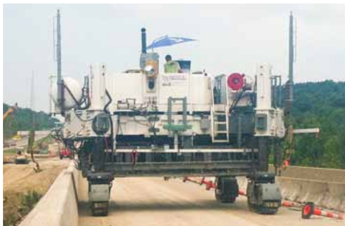
S850SL utilizing SmartLeg and AccuSteer to cross a bridge deck
