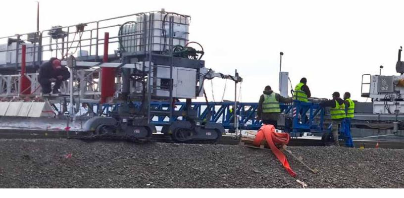
and river washed 'brown sand' while the 7cm (2.75") upper layer uses higher quality crushed aggregates. Both the top and bottom mix concrete is prepared at a nearby batching plant which is run by Heidelberg Cement.
