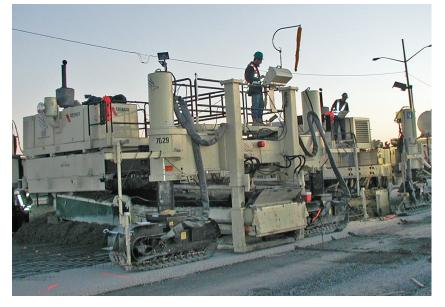
As an option, an additional operation platform with telescopic access walkway can be located on the bolster over the top of the conveyor skip for optimum view of all the machine's dumping and spreading functions. Control Console can be relocated anywhere along the Operator Platform to match operator's preference.
