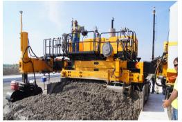
G&Z's powerful concrete spreader plow is easier to change width than an auger. The spreader cart track sections are structural, eliminating the need for intermediate track supports.
